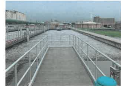
Industrial Aeration Basin
