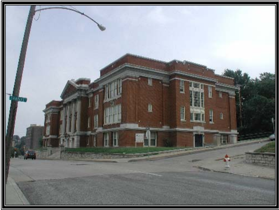
Robidoux School Apartments
