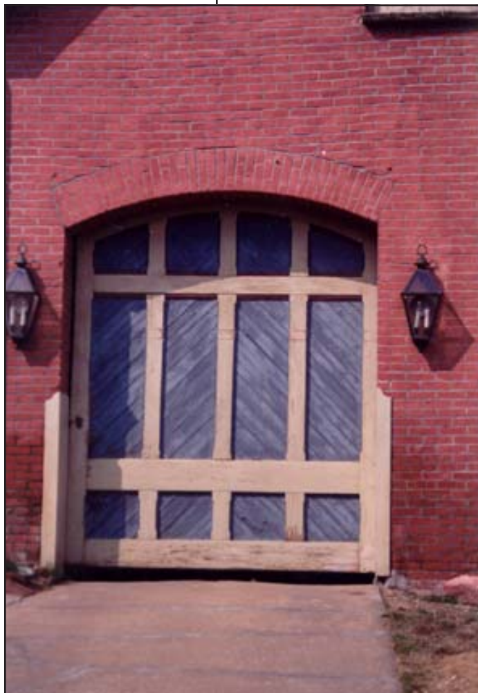
Chamfered stiles, rails and beaded board panels are common elements of late 19th century carriage house doors, as seen here at the Nelson-Riley Carriage House, 605 N. 5th Street, Robidoux Hill Historic District.
