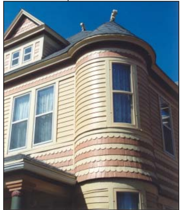
Wood clapboard siding, decorative shingle beltcourses, and dormer gable ornamentation embellish the exterior of the George Schneider house, 1921 Francis Street, Harris Addition Historic District.
