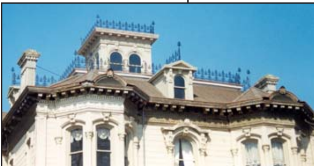
Ornamental iron cresting embellishes the main roof, cupola and dormers of the Adam Schuster Mansion, 703 Hall Street, Museum Hill Historic District.
