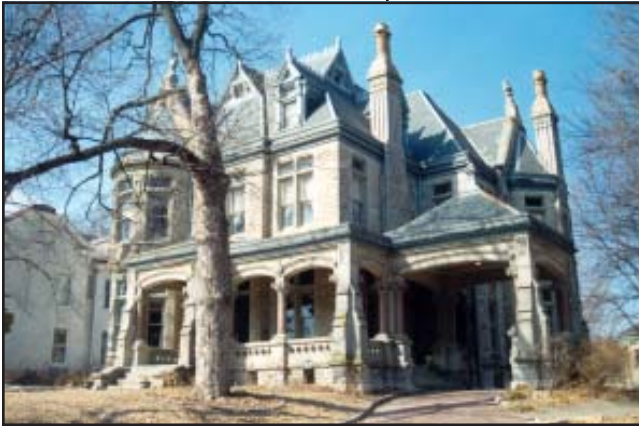
A significant character-defining feature of the Nathan Ogden house, 809 Hall Street, Hall Street Historic District, is its multiple hipped roof complete with slate sheathing, copper ridging, cresting, dormers, stone finials, and towering corbelled chimneys.
