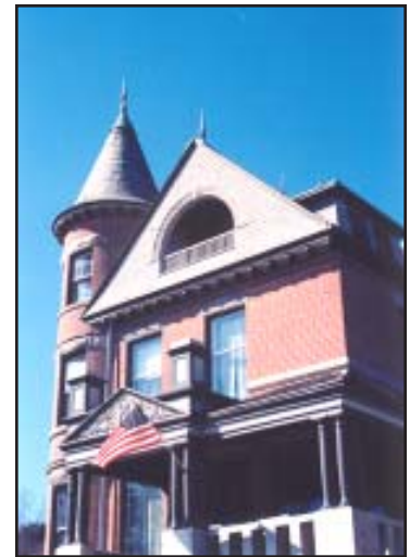
The rehabilitation of the Krug-Hill Mansion, 1105 Krug Park Place, has been one of St. Joseph's most celebrated residential historic preservation projects.
