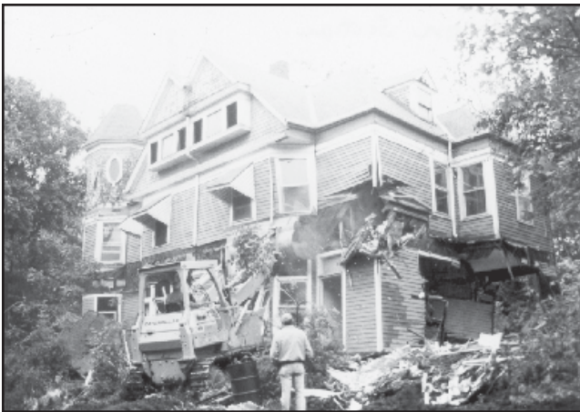
Demolition of the John D. Preston house, 3015 Felix Street.
