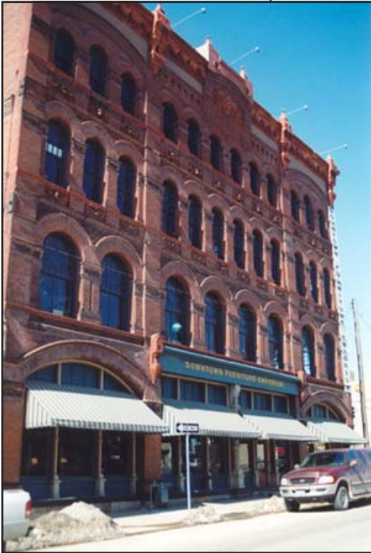
In commercial buildings with traditional storefronts, signs are often positioned on a sign board frieze located above the first floor display windows.
