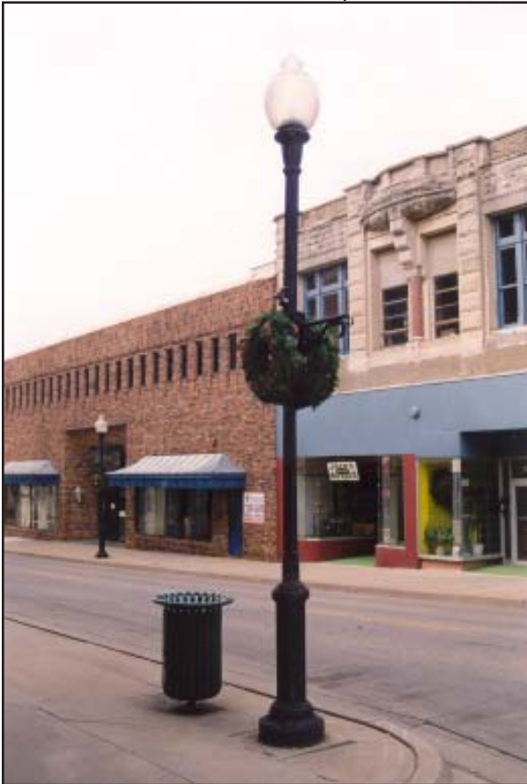
New ornamental streetlights help to enhance the visual quality of Downtown St. Joseph's streetscapes.
