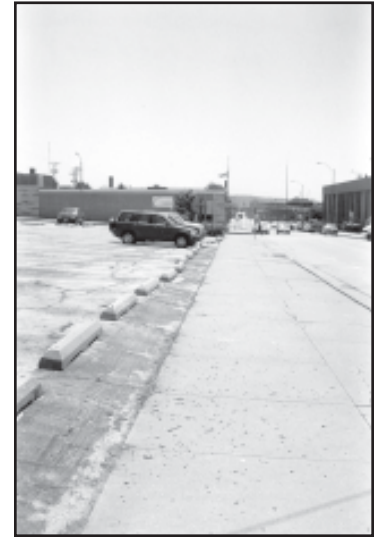
Parking lots such as this one found on 7 th Street in Downtown St. Joseph, are too often characterized by large expanses of concrete with no plantings or screening at their edges to soften their presence in the streetscape.
