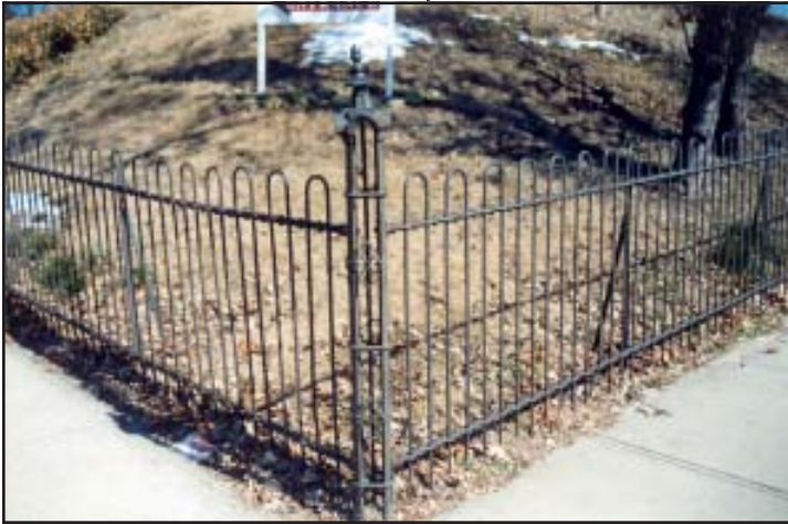
This cast iron fence in a hairpin design is located around the grounds of the former Wyeth-Tootle mansion, now the St. Joseph Museum, 1100 Charles Street, Museum Hill Historic District.
