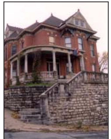
Many of St. Joseph's Victorian residences incorporated elaborate stone carvings and staircase railings into ashlar stone retaining walls to define their entrances.
