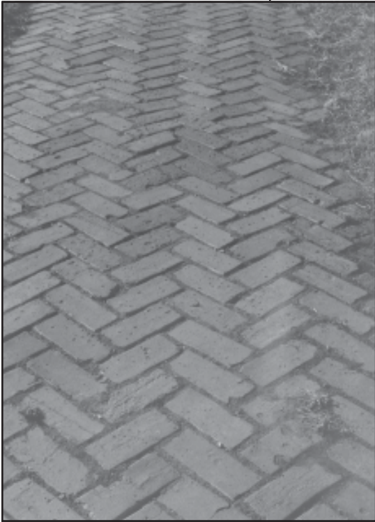
Herringbone-patterned brick sidewalks are common historic landscape features found in many of St. Joseph's historic districts.
