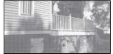
Deck railings, skirtboards, foundation piers and foundation infilling should tie the deck to the house in a similar manner as a porch.
