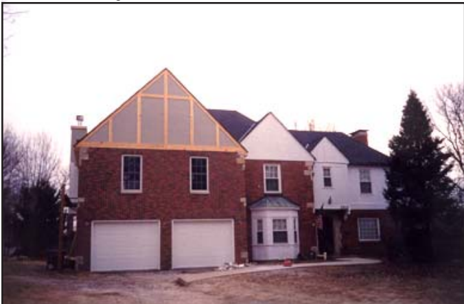
A new addition with two-car garage is added to this 1930's Tudor Revival style home on Lover's Lane with a sensitive eye to the original building's style and detailing.
