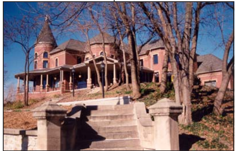
The completed Victorian Revival mansion built at 520 S. 11 th Street, Museum Hill Historic District, rises majestically from its corner lot and pays homage to the neighborhood's high style Victorian heritage.
