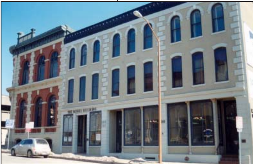
Rehabilitation of historic commercial buildings reinforces the character of St. Joseph's downtown.
