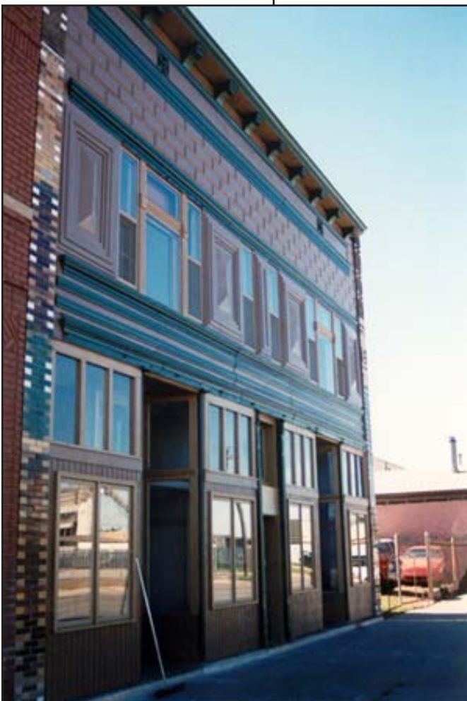
The 1905 Burnette-Leibowitz building at 819-821 S. 8th Street has a rare surviving stamped metal facade.
