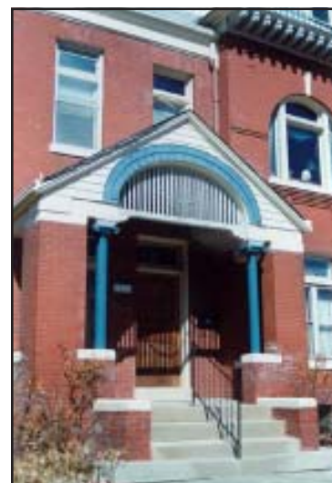
The entrance porch of the Louis C. Burnes house, 1923 Francis Street, Harris Addition Historic District.
