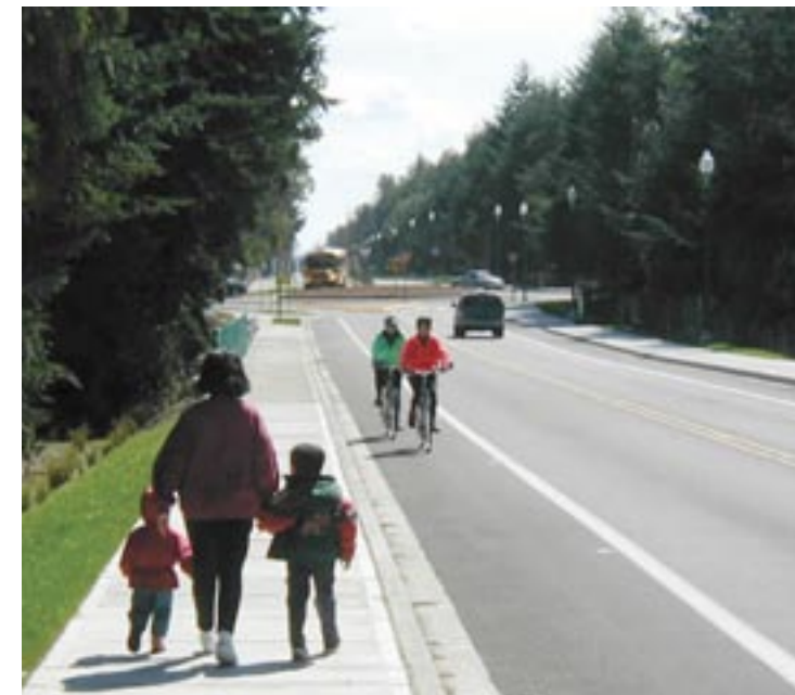
Lower volume, but direct routes may be suitable for dedicated bicycle and pedestrian connections. In this case, the bicycle lane provides a buffer between moving vehicles and the sidewalk. Street lights emphasize the importance of this route to the community. (Source: Photo courtesy of Dan Burden, Complete the Streets Coalition).
